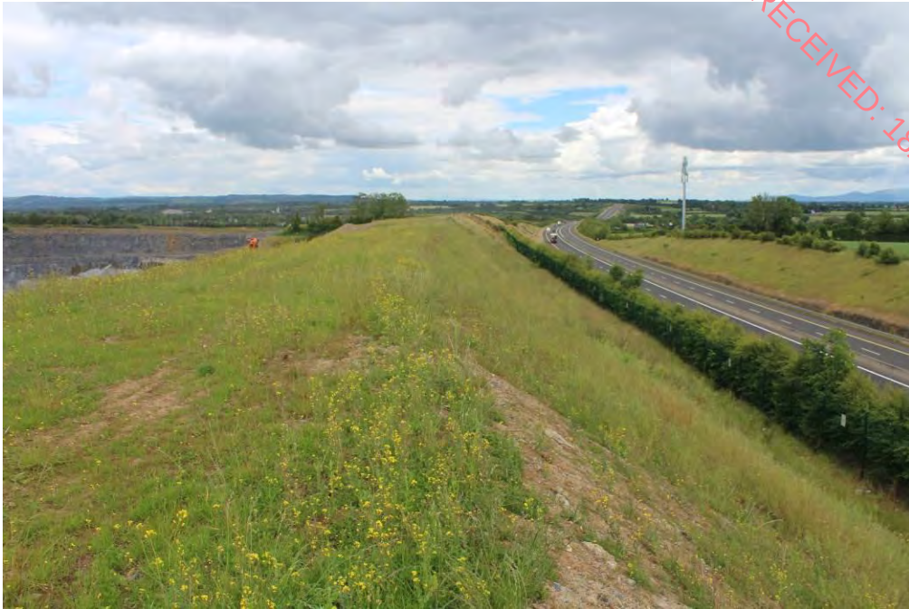
Figure 13 Bund running along southern boundary of the quarry
