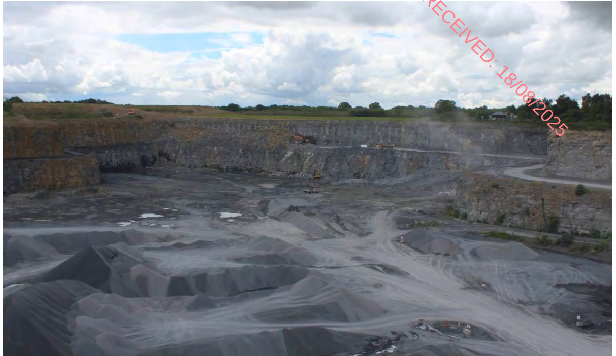
Figure 31 South Western face
