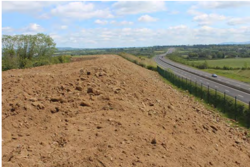
Figure 40 Bund on completion
