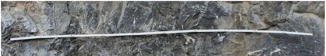
Upper North Western Face: Unweathered, medium thick bedded limestone. Medium joint spacing. Low joint aperture with some light brown staining. RQD-88.
