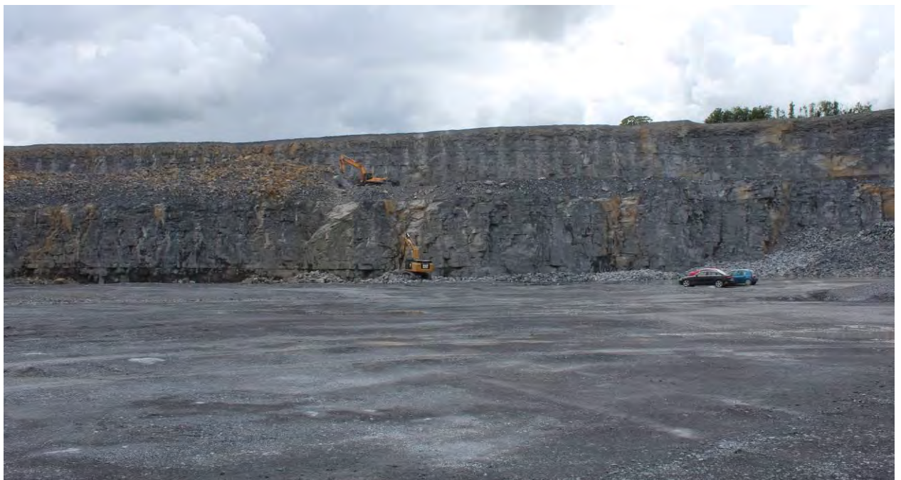
Figure 10 The new south western side of quarry all benches under 20m in height
