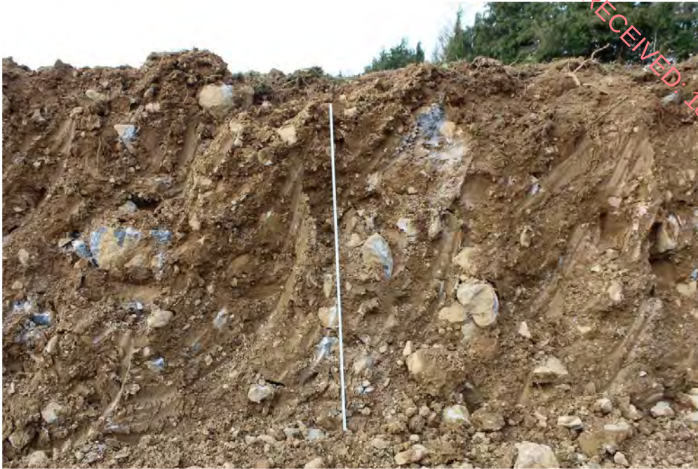
Figure 37 Excavated material used in bund construction
