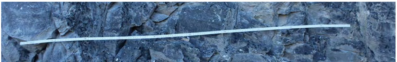
Upper North Western Face: Unweathered, medium thick bedded limestone. Medium joint spacing. Low joint aperture with some light brown staining. RQD-78.
