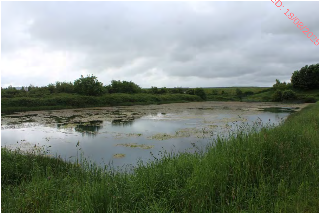
Figure 14 Showing larger settlement lagoon
