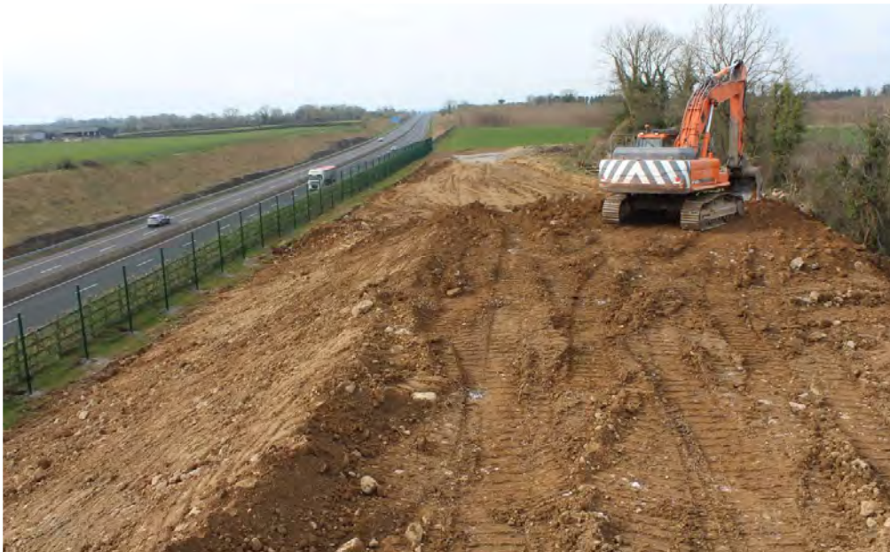
Figure 38 Bund Construction
