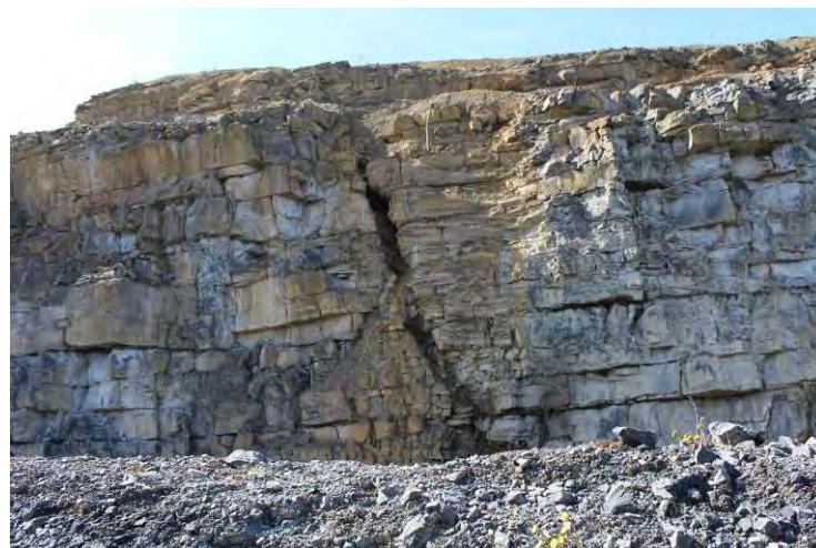
Figure 5 The main West East trending fault in the northern portion of the west face
