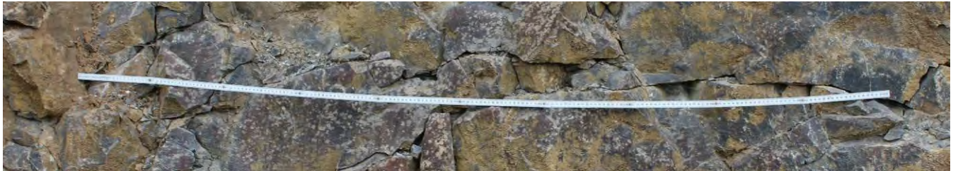
Middle North Western Face: Minor Weathering, medium thick bedded limestone. Medium to large joint spacing. Low joint aperture with orange staining. RQD-86.
