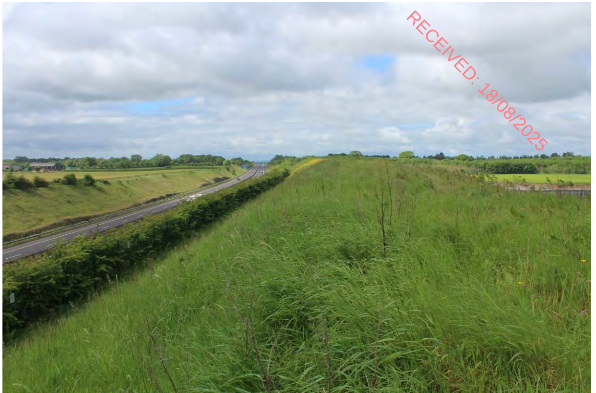
Figure 12 Bund on southern side of quarry.
