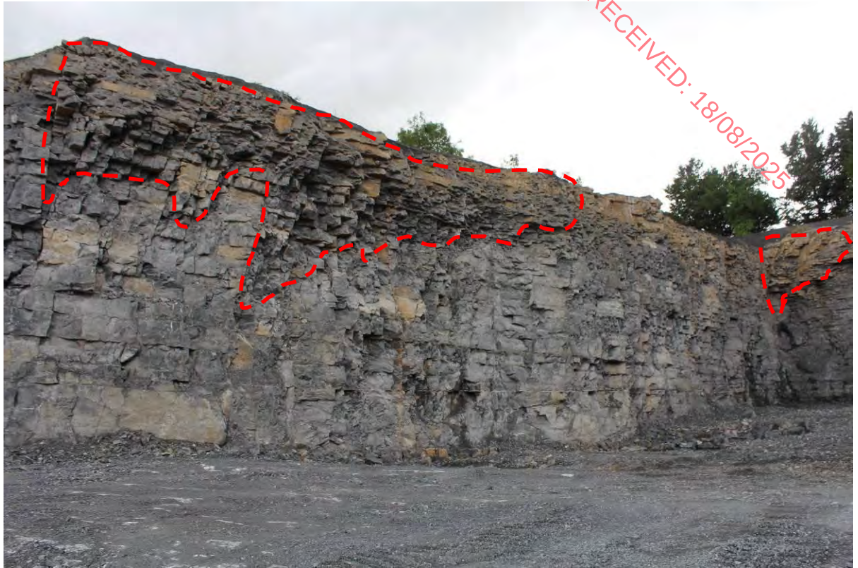
Figure 33 Overhang in south west corner
