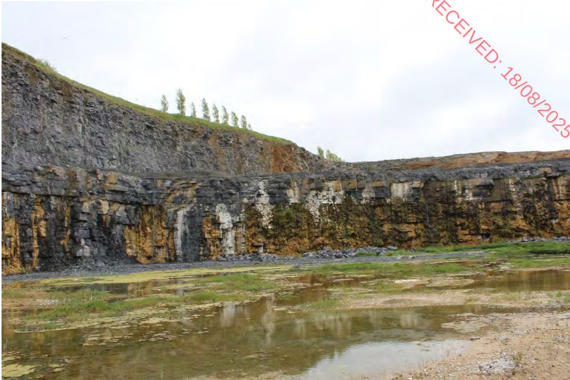
Figure 28 Eastern Lower Face water infiltration
