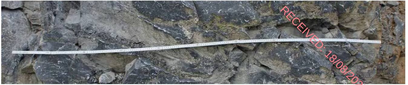
Upper North Western Face: Minor Weathering, medium thick bedded limestone. Medium to large joint spacing. Low joint aperture with some light brown staining. RQD-84.
