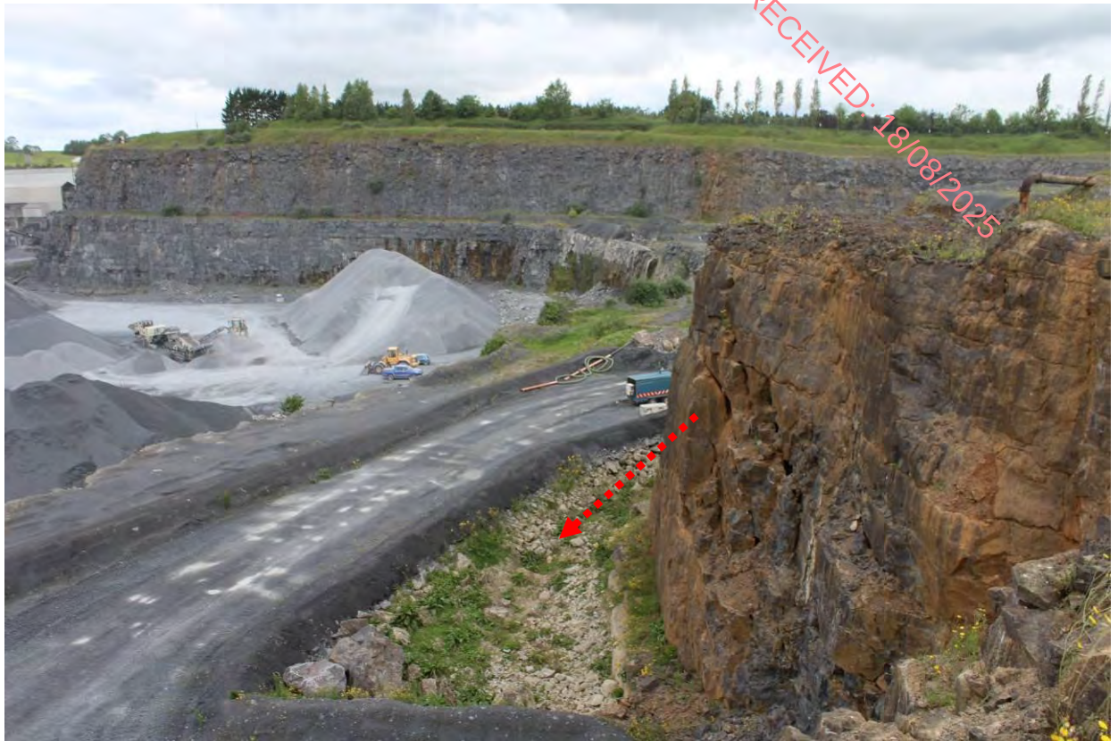
Figure 21 Loose Material in Eastern upper face
