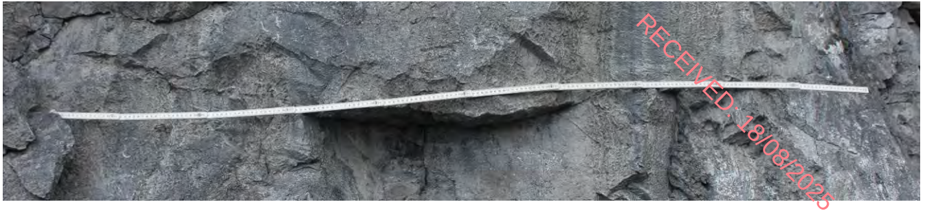
Upper South Western face: Unweathered, medium thick bedded limestone. Large joint spacing. Low joint aperture with clean joint surface. RQD-92.
