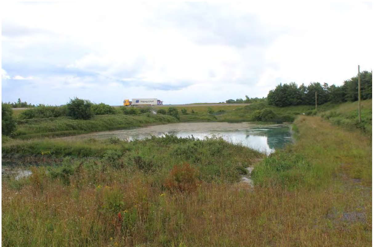
Figure 15 Showing larger settlement lagoon
