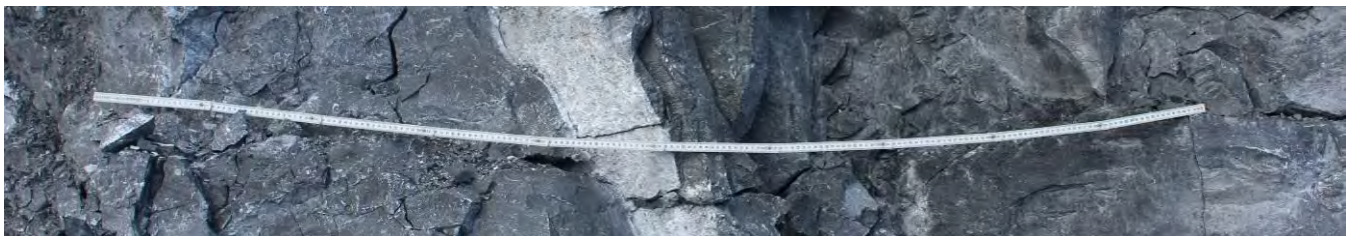
Lower South Western face: Unweathered, medium thick bedded limestone. Medium joint spacing. Low joint aperture with some light calcite infill. RQD-80.
