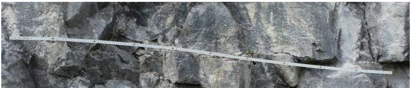
Middle South Western face: Unweathered, medium thick bedded limestone. Medium joint spacing. Low joint aperture with clean joint surface. RQD-82.
