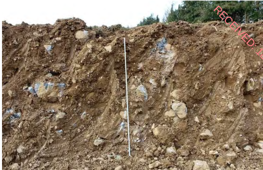
Figure 35 Excavated material used in bund construction
