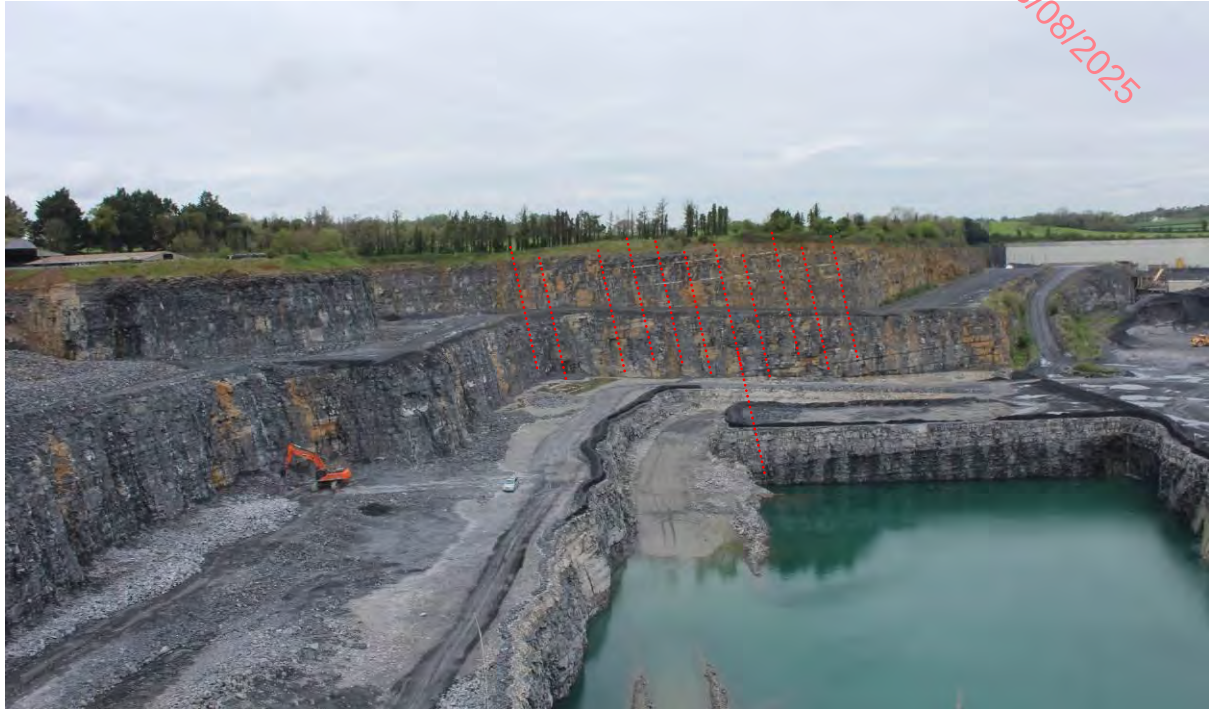
Figure 6 The Primary joint set (highlighted in red)
