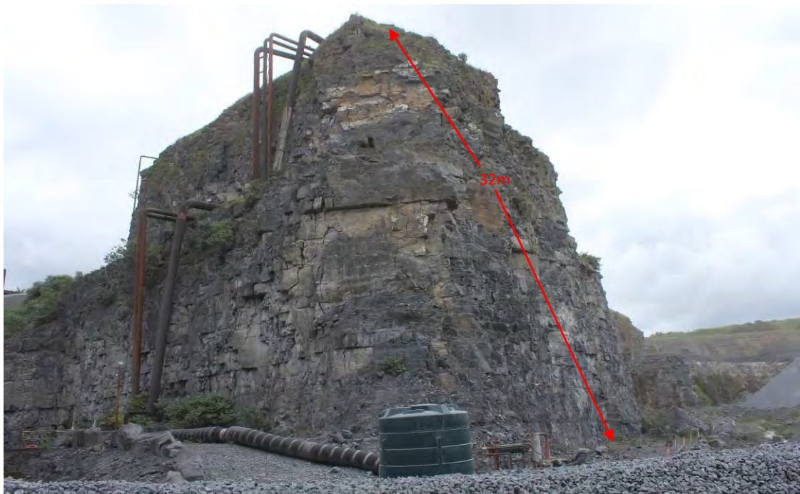
Figure 23 Eastern Upper face showing decreasing middle bench width
