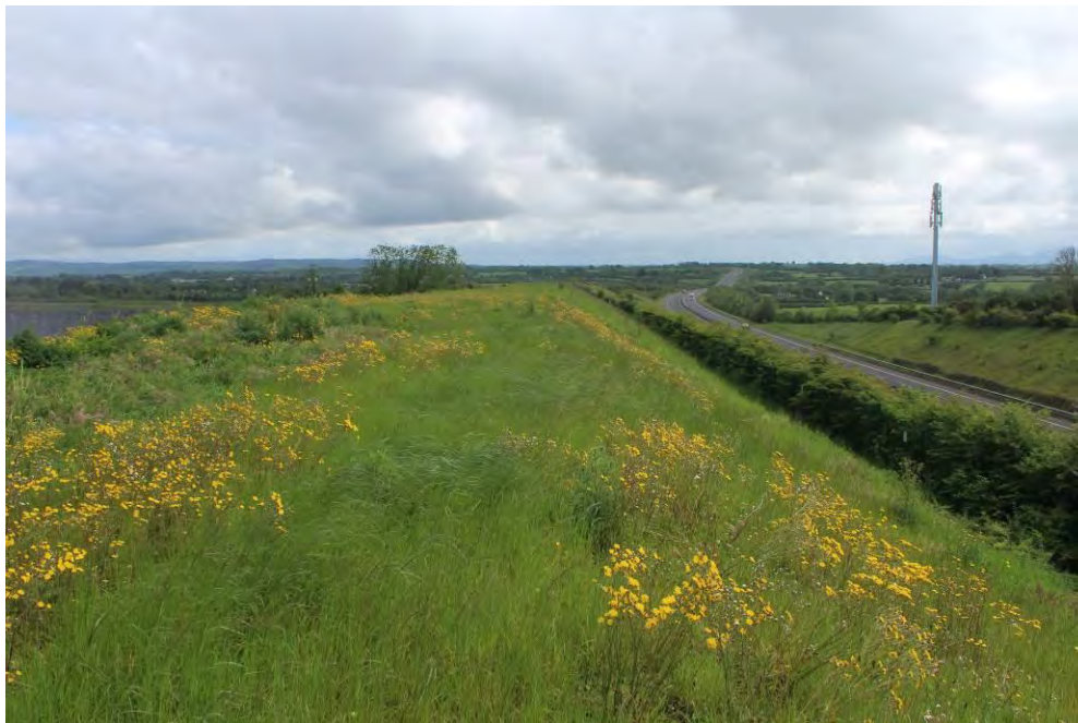
Figure 38 Bund on completion and bund in 2024
