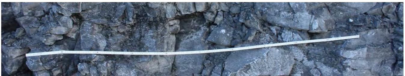
Upper North Western Face: Unweathered, medium thick bedded limestone. Medium joint spacing. Low joint aperture with clean joint surface. RQD-76.
