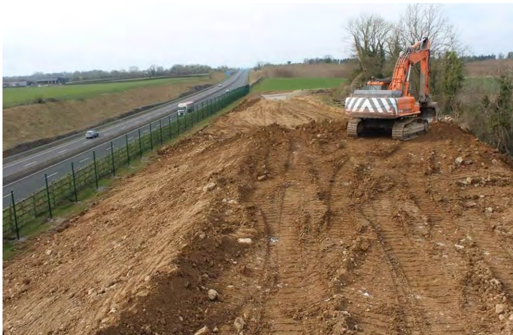
Figure 36 Bund Construction
