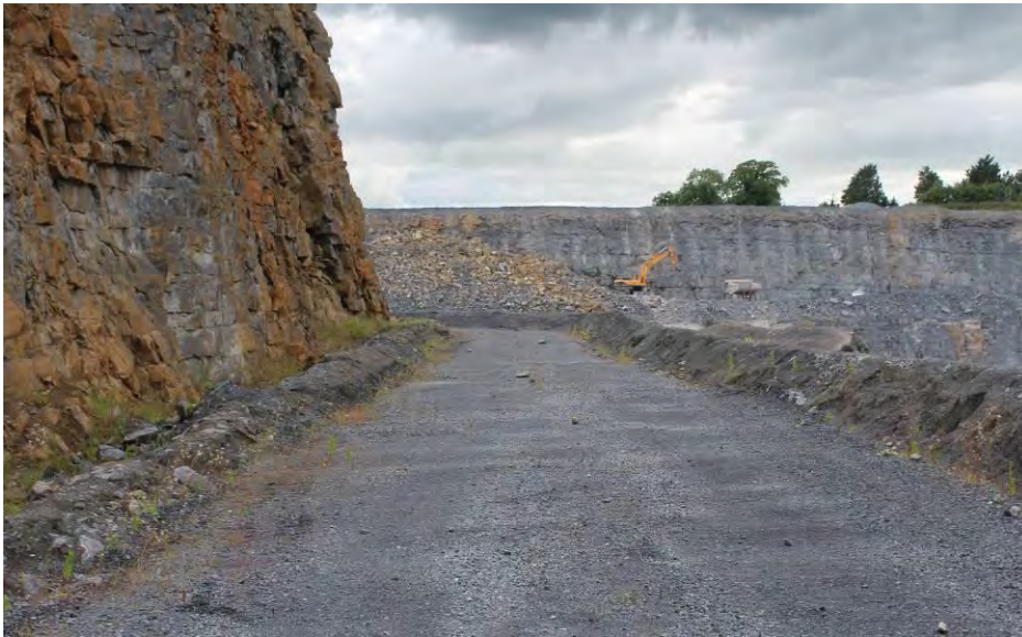
Figure 18 Southern Upper Face weathered section and evidence of small loose rock
