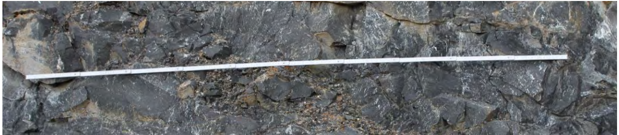
Figure 20 RQD of Southern Upper face
