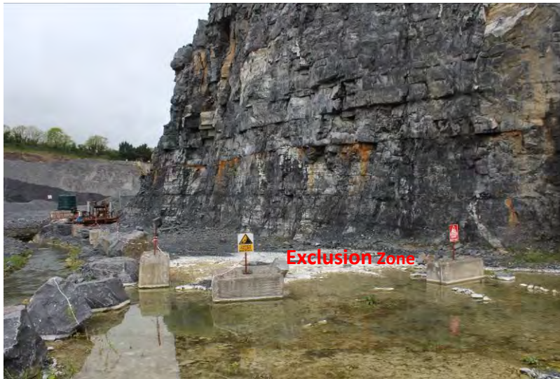
Figure 25 Exclusion zone beneath overheight face.
